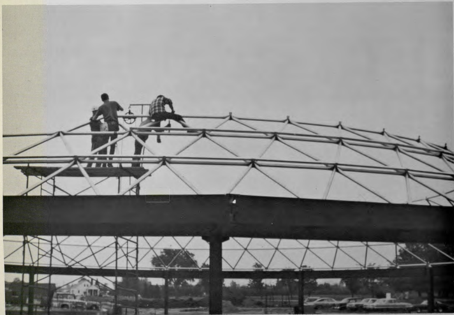
Figure 6 - Cantilever Erection Method on Dome Roof.
