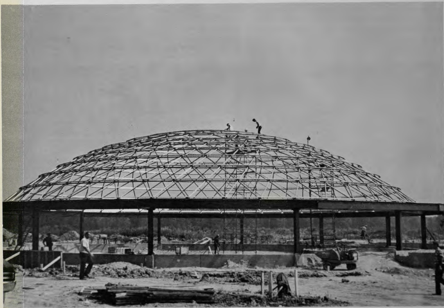
Figure 2 - Reticulated Roof (Courtesy of Butler Manufacturing Company).
