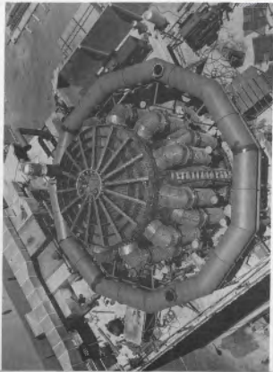
Figure 3. BTKM Building with Chamber in Place (upper building being fabricated)
