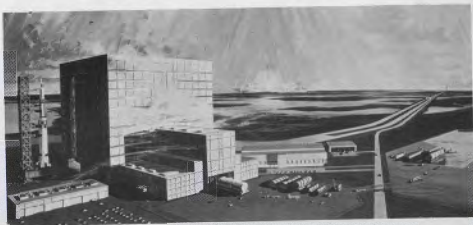
Figure 12. Complex 39, under construction for NASA, will become the Nation's Moonport.
