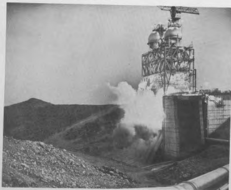
Figure 2. F-1 Engine Undergoing Static-Test on Stand Constructed by Corps of Engineers
