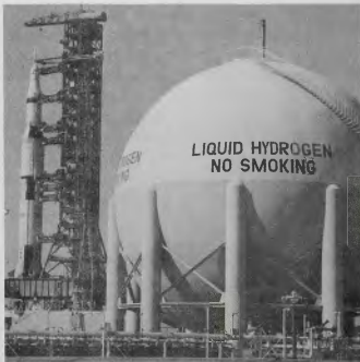
FIGURE 11 - LIQUID HYDROGEN STORAGE SPHERE
