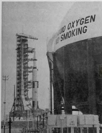
FIGURE 14 - LIQUID OXYGEN STORAGE SPHERE
