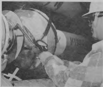
FIGURE 35 - INSPECTOR CHECKING THE INTERPASS TEMPERATURE ON A WELD IN VACUUM JACKETED PIPING
