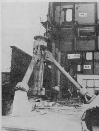
FIGURE 3 - HANGING GIRDER G-14
