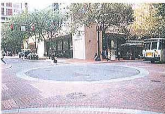
Pavers at intersections signify importance of location and aid in traffic safety by slowing traffic and designating crosswalks.
