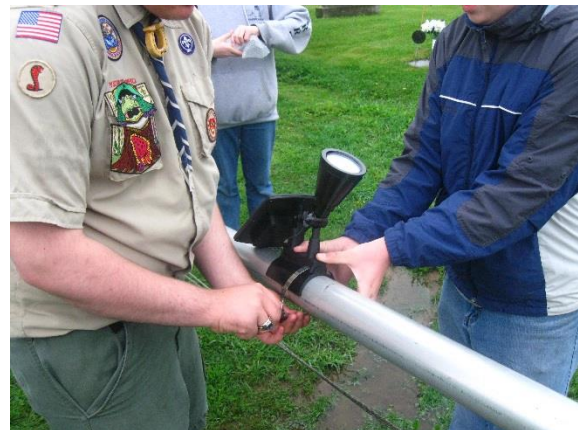
Solar light being installed on the flagpole at Cushing Cemetery
