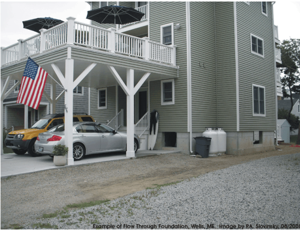
Example of Flow Through Foundation, Wells, ME. Image by PA. Slovinsky, 08/2008
