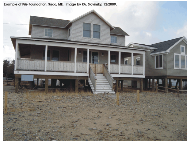
Example of Pile Foundation, Saco, ME. Image by PA. Slovinsky, 12/2009.
