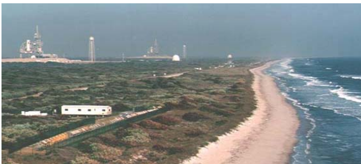
Figure 1. KSC's Beach Corrosion Test Site
