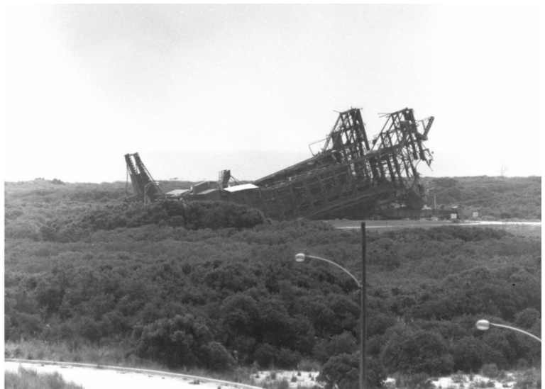
Figure 3 - Service Tower Demolition, 1976
