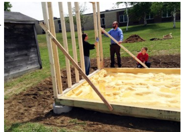
Greenhouse construction (photo courtesy Sally Allen)
