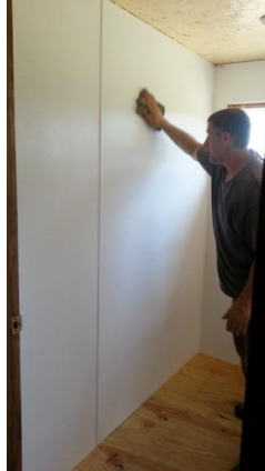
Dana Rogers working on the Grange bathroom Photo by Debbie Rogers
