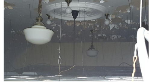
Above suspended ceiling in the grange Photo by Dana Rogers Jr.
