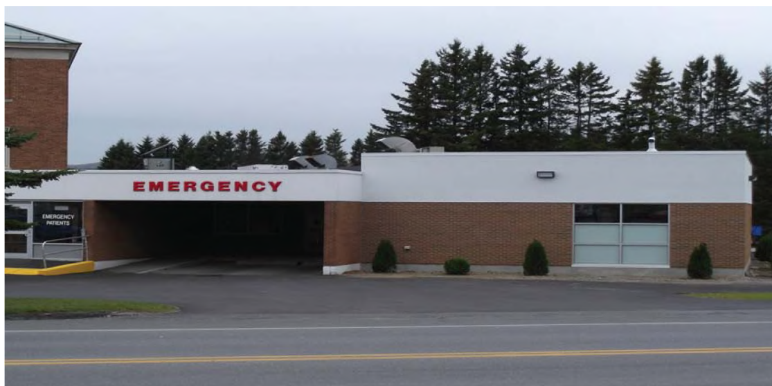
Northern Maine Medical Center built a new addition for the MRI.
