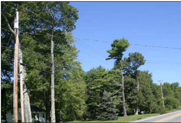
Figure 2-37 Above ground utility lines are less visible
