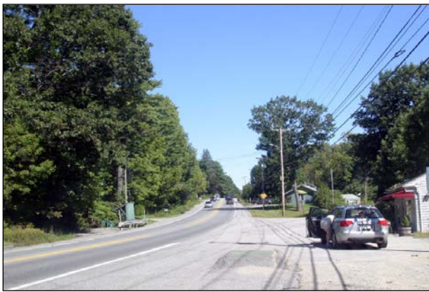
Figure 2-26 View north entering the Village 2 District transitional zone
