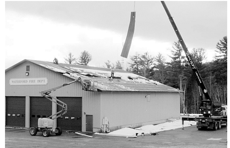
Strong winds Nov. 2 rolled up the roof over the fire station. All of the metal roofing on the north side had to be removed. The project was completed Dec. 5.
