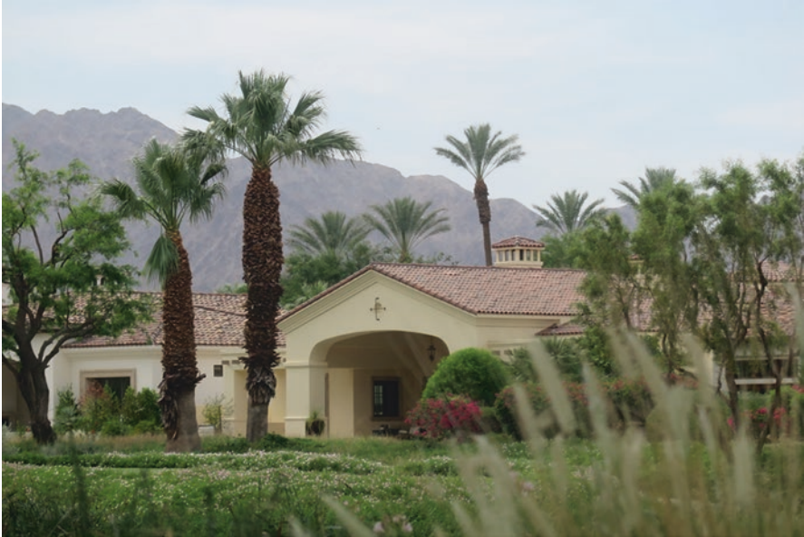
Fig. 7.3 Residence impacted by IID's Cessation of Net Metering, at Trilogy at the Polo Club, Indio, CA
