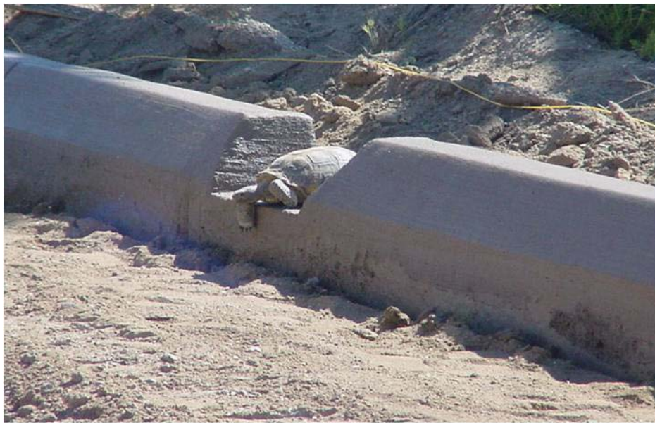
Figure 2-1: Tortoise in Tortoise Trot (asphalt not poured in road yet)
