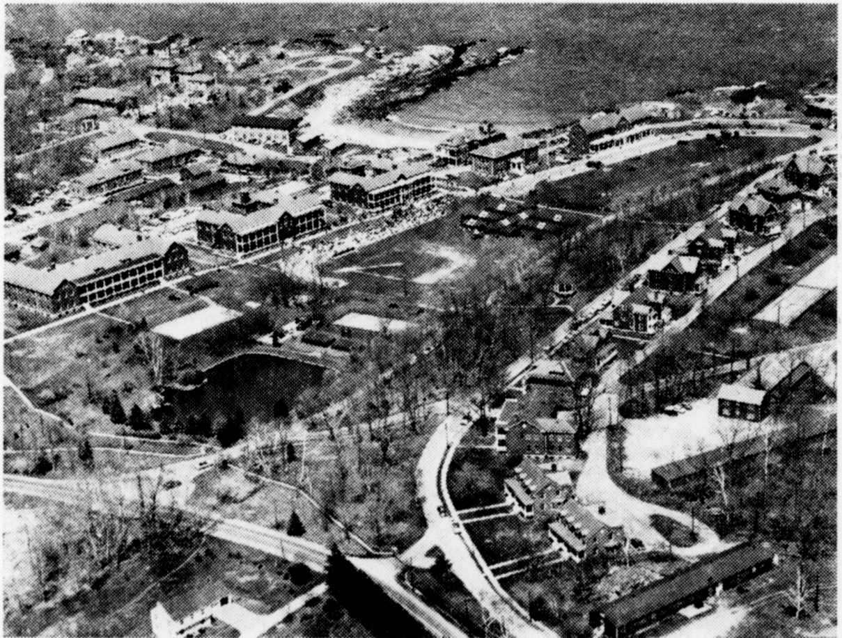
Aerial view of Fort Williams at Cape Elizabeth
