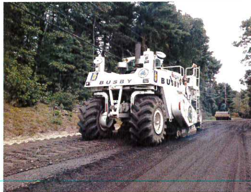
Reclaiming on Anderson Road and Windham Center Road.
