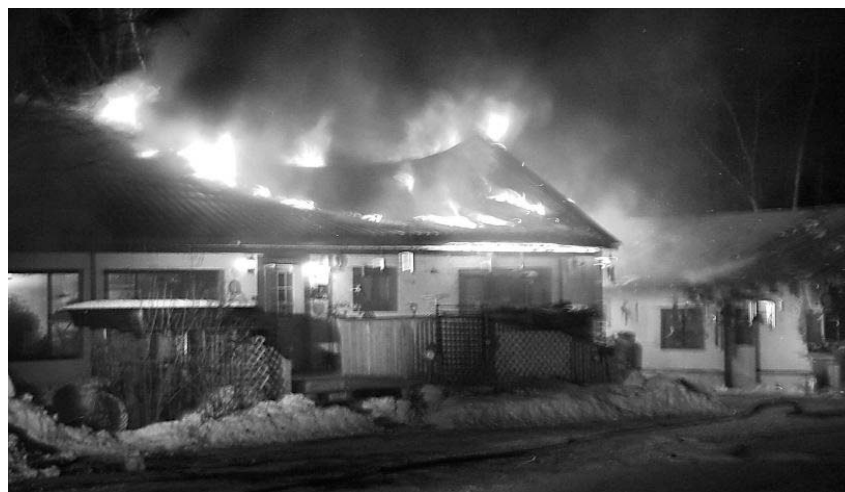
Fire broke out at the David Hart and Rockie Graham home in Just Rite Acres around 5 p.m. Dec. 23 when sliding ice knocked a metal chimney off the roof, allowing wood stove embers to ignite roof timbers. Waterford Fire along with three neighboring departments brought the fire under control. The occupants, home at the time, escaped unharmed.
