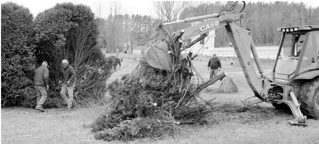
ELM VALE REMOVAL- Members of the Waterford highway crew removed three overgrown cedar bushes from the town-owned Elm Vale Cemetery Dec. 7. Bill Murch and Albert Heath work at left while Road Commissioner Brad Grover observes Miles Millett operate the backhoe.
