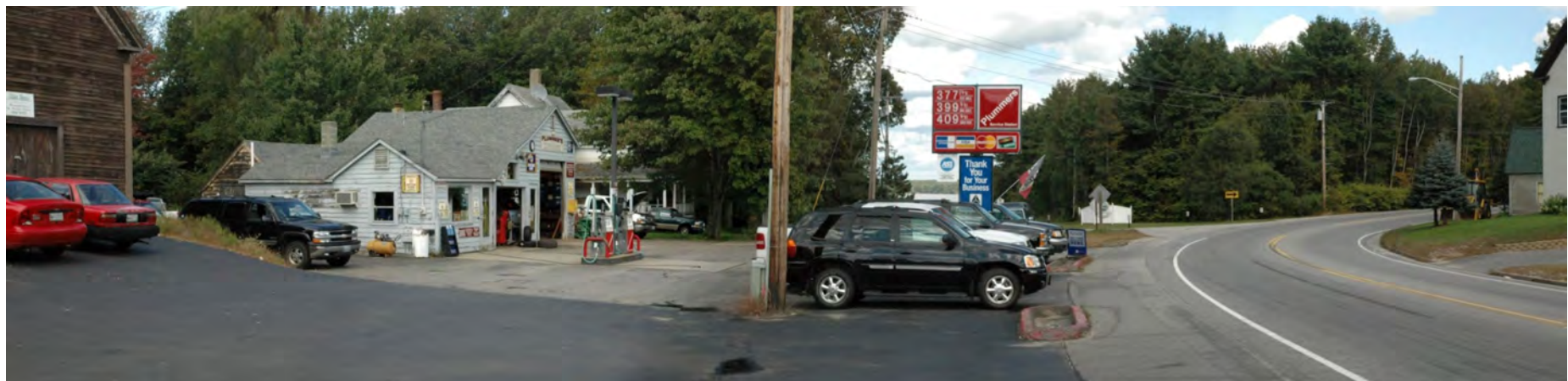
A new sidewalk within the Route 35 ROW would strengthen the relationship between the Village Core, the lake, and Johnson Field.
