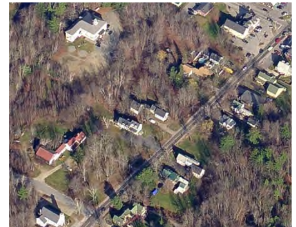
Aerial view of Route 35 south of the Village Core.
