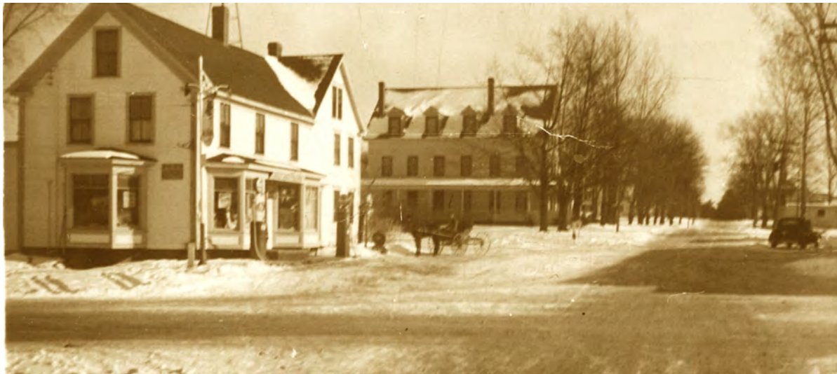
Looking east from the intersection of Routes 35/114 at the turn of the century.
