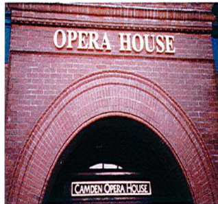
The use of raised gilded letters complements a classic building and produces a highly legible sign.
