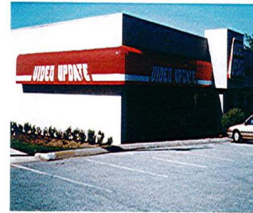
An awning used as an advertising feature and sign, which would be inappropriate on most downtown buildings.
