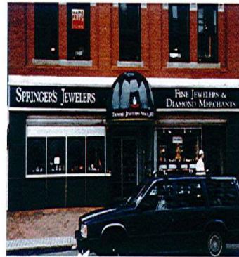
An awning used to emphasize the entrance of the building and provide some measure of shelter.
