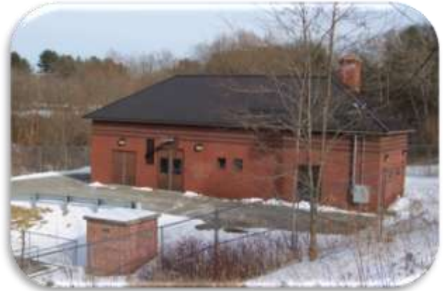
Bear Brook Pump Station
