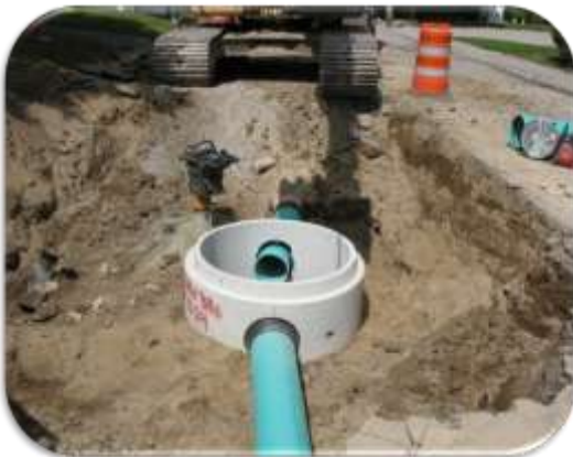
Installation of a new manhole on Pleasant Street
