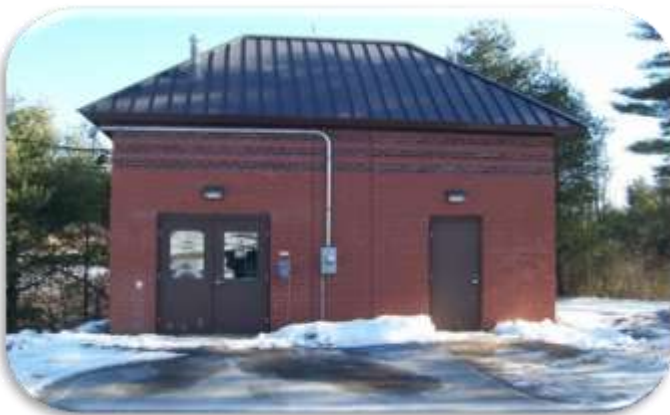
Millbrook Pump Station
