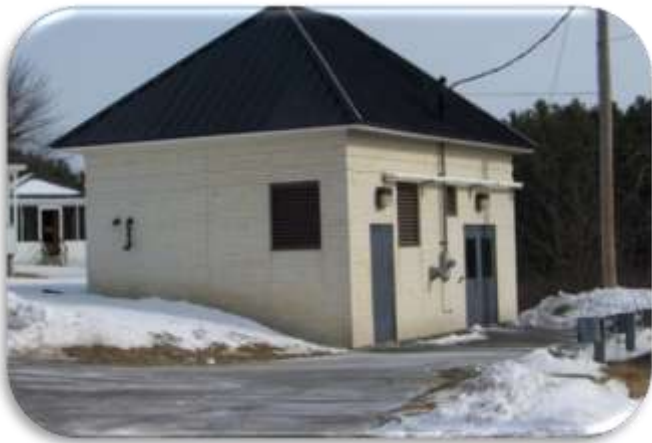
Goosefare Pump Station
