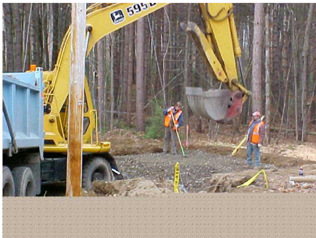
WORKING ON THE NEW SEPTIC SYSTEM AT THE NORTH STATION
