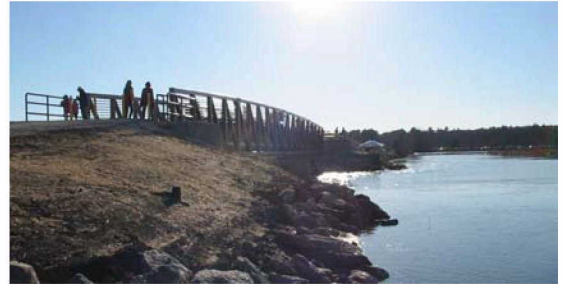
New Scarborough Marsh Eastern Trail Bridge
