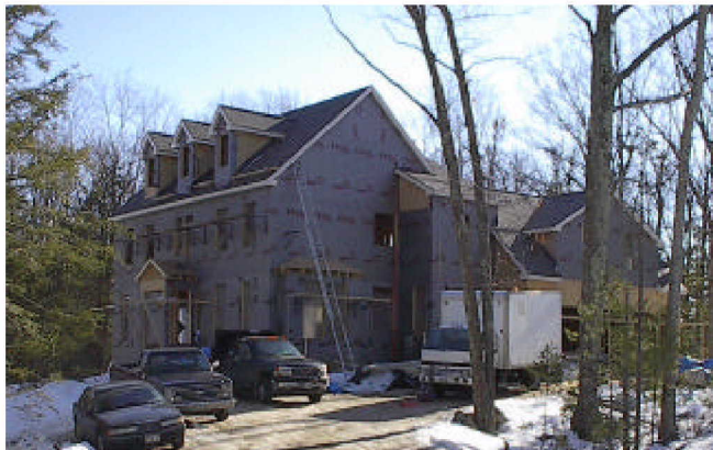
Home under construction, Plymouth Drive
