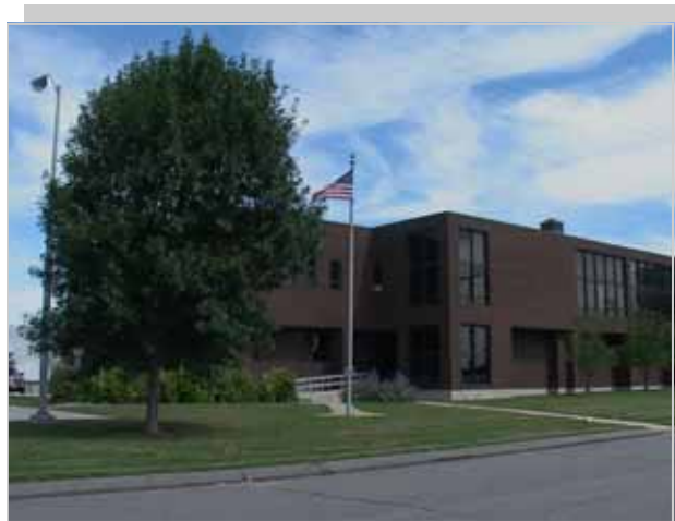
Water Resource Protection, Waterman Drive
