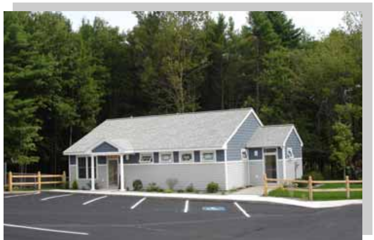
Collection Systems Division Office Building
