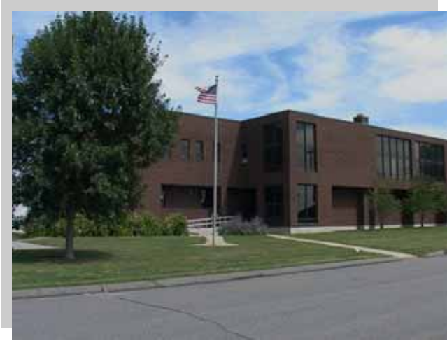
Water Resource Protection, Waterman Drive
