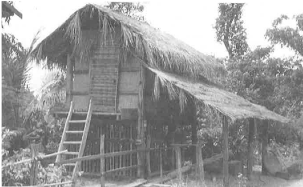
Houses on stilts in Vang Village stayed dry during the rainy season.
