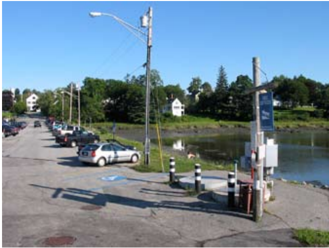
A view of the array of infrastructure in the study area: utility lines and poles, transformers, lighting, the boat launch, the pump station and manhole covers for the force main and the outfall. The Great Salt Bay Sanitary District easement runs straight down the aisle of parking. Just beyond the pump station in the rip rap below the park are three stormwater outfalls
