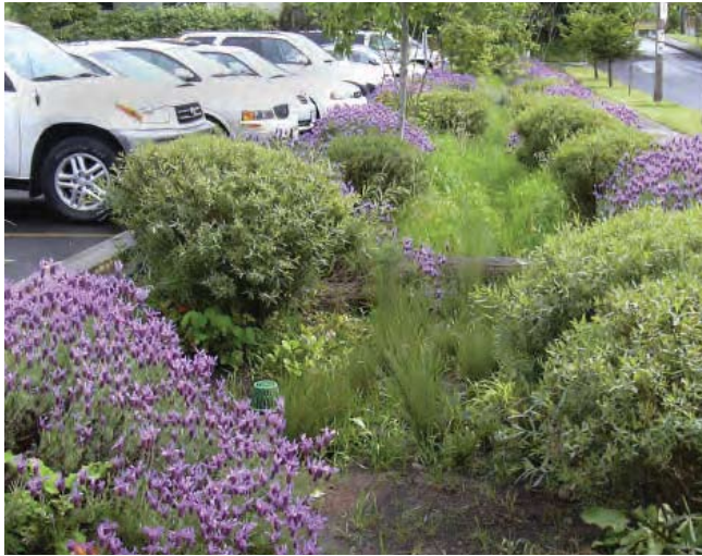
Example of a rain garden / bio-swale. Courtesy Stormwater Solutions Handbook, Portland OR
