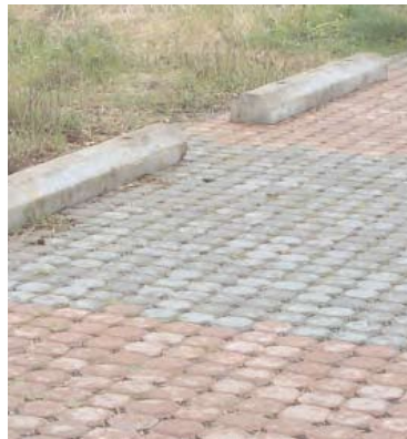
Example of pervious pavers in a parking lot. Courtesy Stormwater Solutions Handbook, Portland OR
