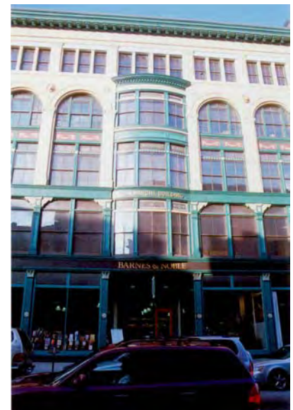
“151 Merrimack Street, Le Bon Marché building and current address of Barnes and Noble Bookstore in Lowell.”
