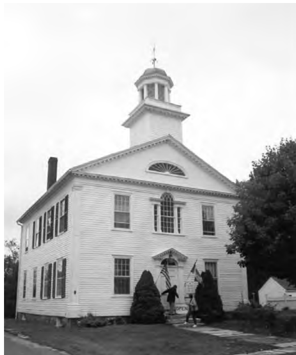
53 Tolland Green, the Old Tolland County Courthouse, where the first floor is the current home of the FCGSC Library. Photo by Albert J. Marceau, Oct. 11, 2006.
