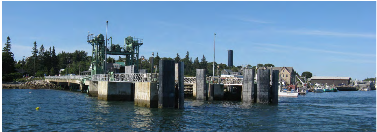
Vinalhaven ferry terminal.
