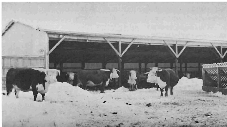
FIG. 2. The open-front pole barn is adequate shelter for beef cattle in Maine. This type of structure is the basis for housing cost information developed for this bulletin.
