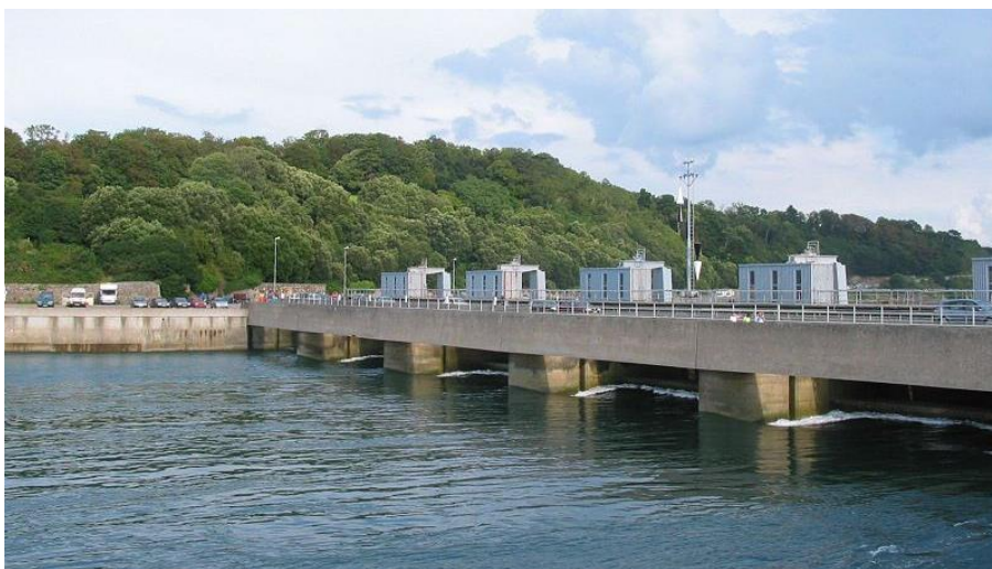
Figure 1.2 – The second largest tidal barrage in the world, La Rance Tidal Power Plant, located in Brittany, France. (Image source: http://www.energybc.ca/profiles/tidal.html )
