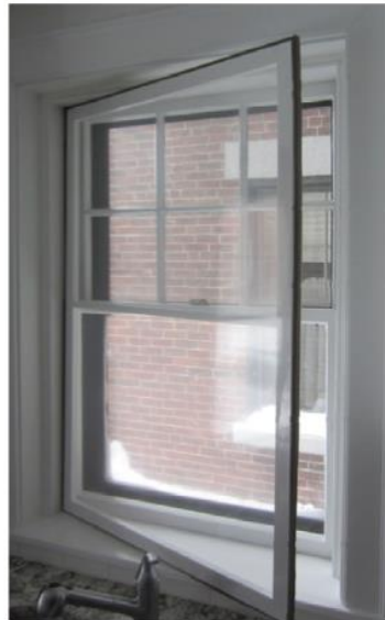
Insert being installed
