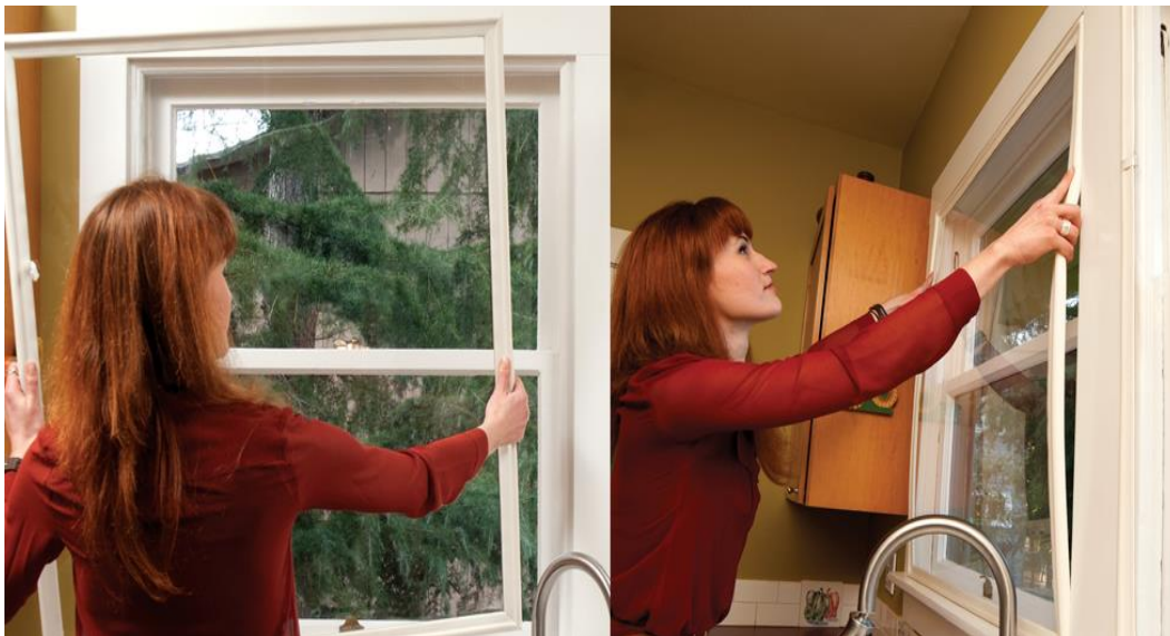
Figure 3 – Indow Window installation process [12]
