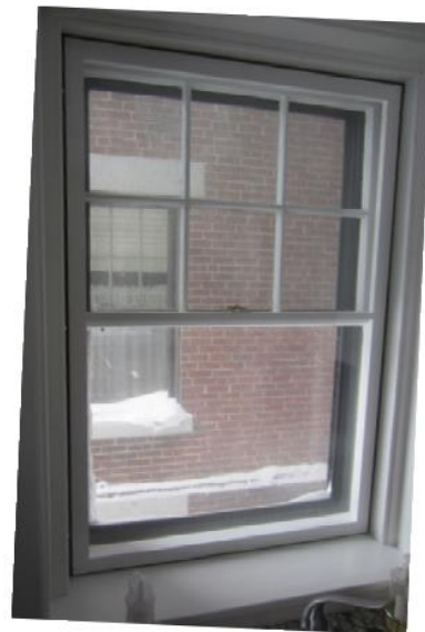
Insert in place
