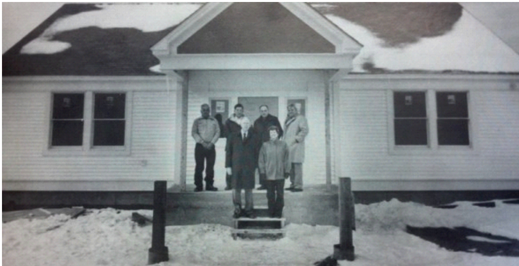
West Bath Town Hall under construction 1989. Pictured are Building Committee members back row left to right: Arthur J. Reno Sr., Willard McCabe, Lewis Atwood, Richard Coombs. Front: Courtney Stover, Kathleen Rogers.
