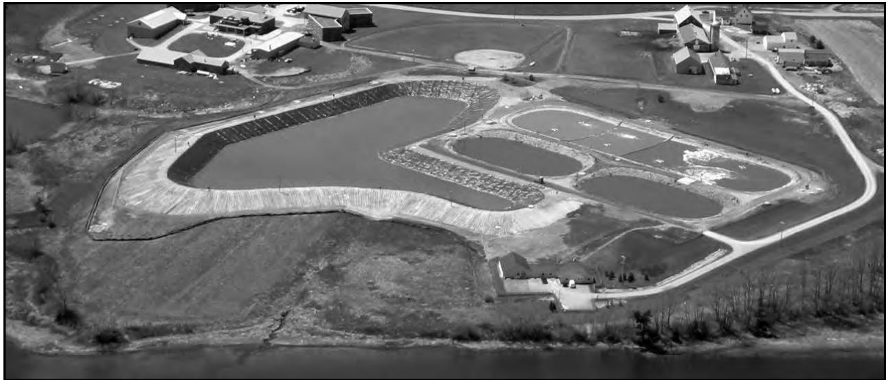
An aerial view of the Warren Sanitary District treatment plant.
