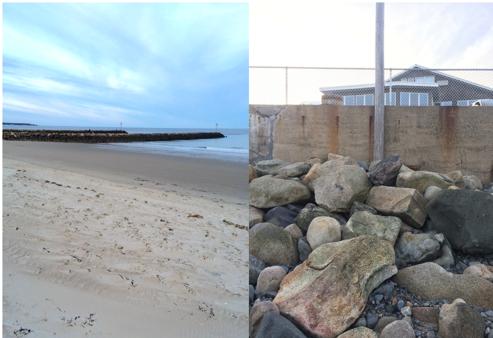
Figure 6. Left, the jetties surrounding the Webhannet River outlet on the northern end of Wells Beach. Right, large boulders front the concrete seawall at the southern (DeVoe, 2016i).
