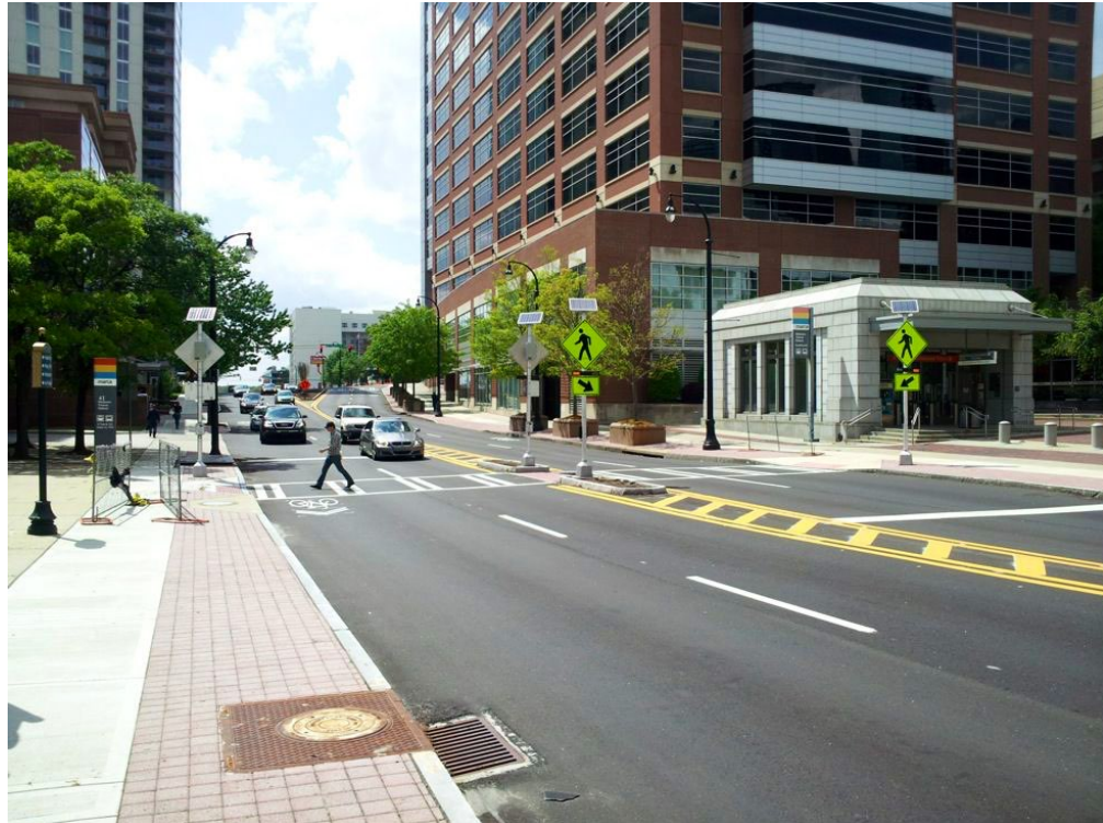
Figure 3.2. Un-signalized pedestrian Crossing (“Midblock Crosswalks - national association of city transportation officials,” n.d.)
