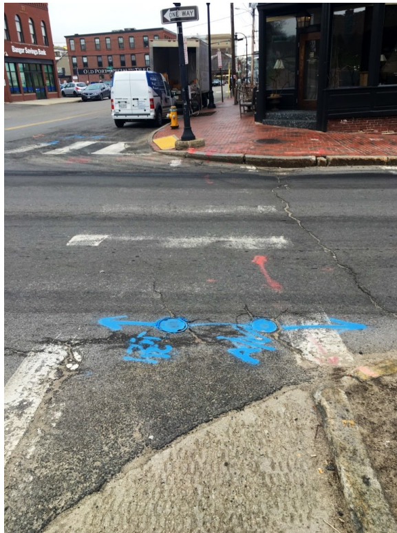
Figure 2.9. Middle Street Crosswalk
