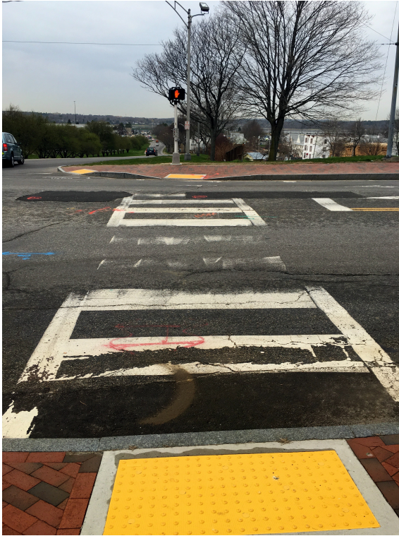
Figure 2.7. Cumberland Street Crosswalk
