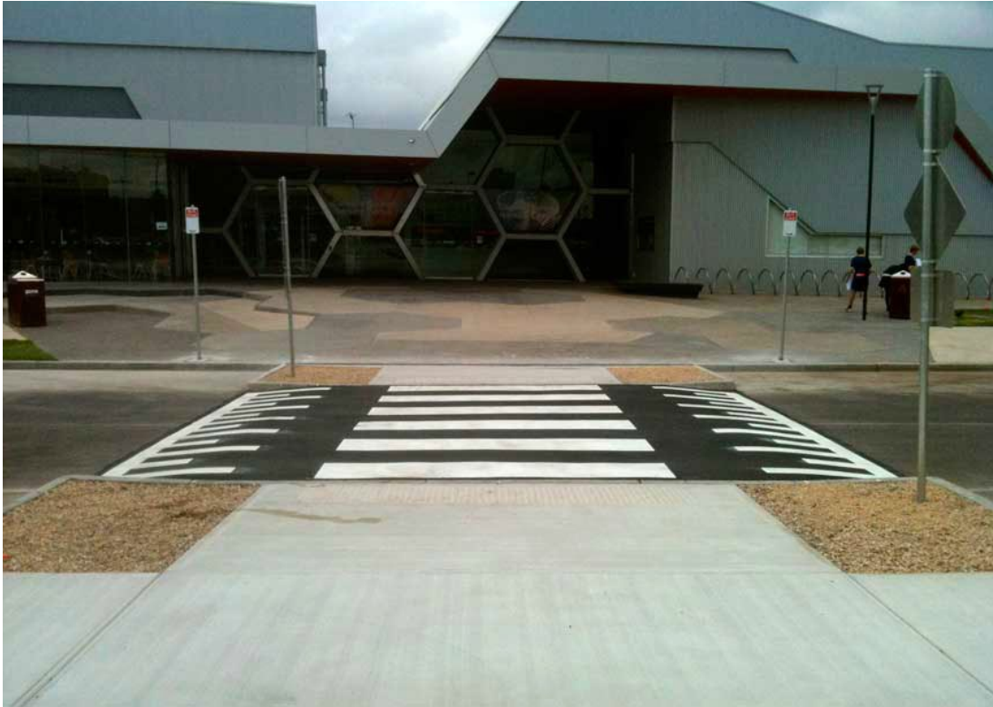
Figure 3.4. Speed Table at Crosswalk (“Western Line Marking,” 1995)
