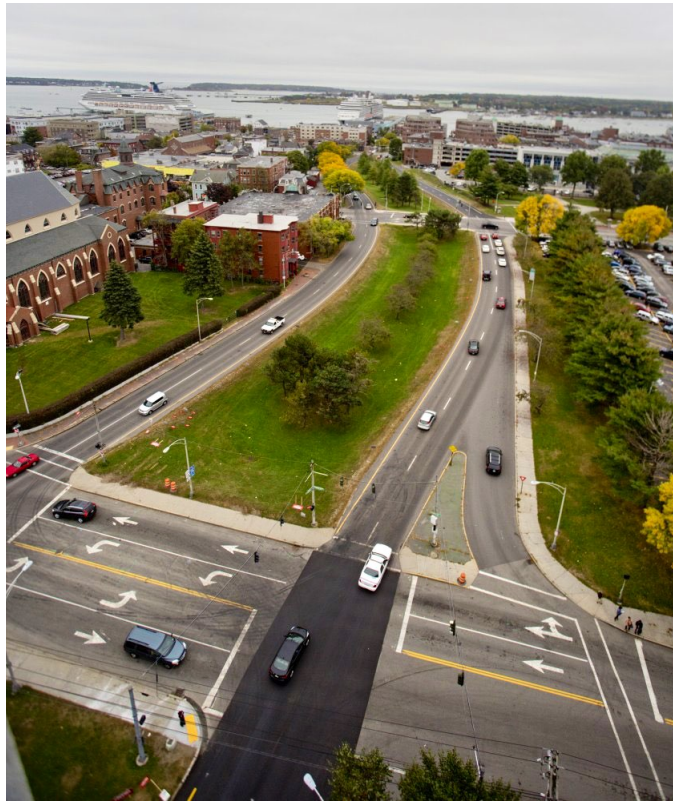
Figure 2.13. Franklin Street Arterial Aerial View (Souza, 2016)
