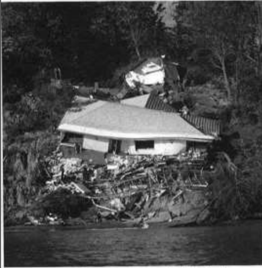
This house was destroyed when the land under it collapsed.
