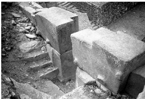
Figure 7: Back of Puerta Principal showing an “ear” on the lower left jamb stone (viewer’s perspective).
