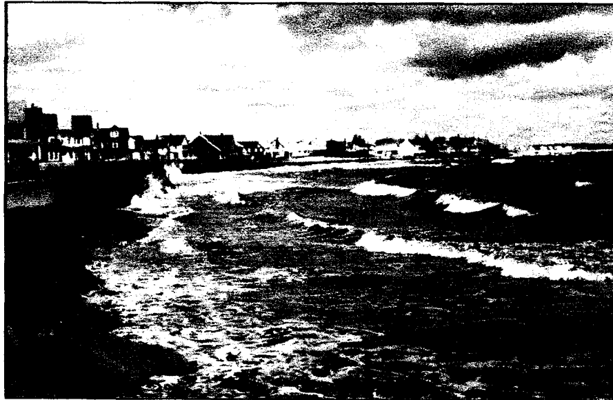
Figure 4.17 Photograph of eroded Wells Beach from 1983. There is very little dry beach and the waves are breaking on the seawalls (Photo courtesy of J.T. Kelley).
