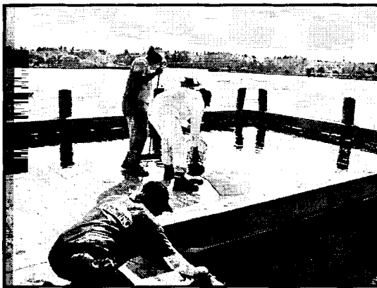
Figure 3.23 First coat of CIM 1000 application and appearance after curing
