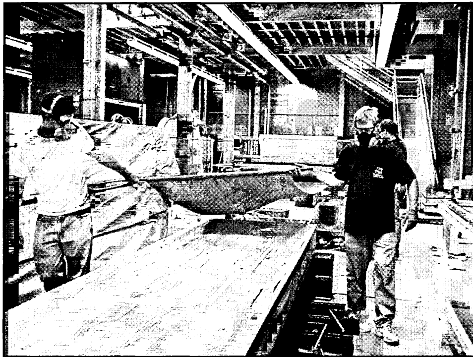
Figure 3.8 Placing the a layer of wet-impregnated glass onto glulam panel for Milbridge Pier
