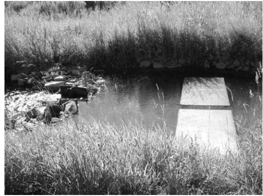
FIGURE 2.—Photograph of the backwatered horizontal flat-plate fish screen (the Malheur screen) and the rock weir flow control structure located in the east canal of the Donner und Blitzen River, Oregon.
