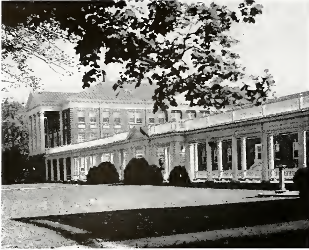
The Colonnade with the Student Building in the background.
