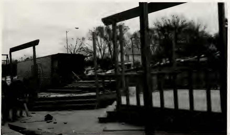
The Lankford Deck — almost completed.
