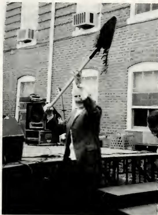
Dr. Healy breaks the ground for the Blackwell Mall Project.
