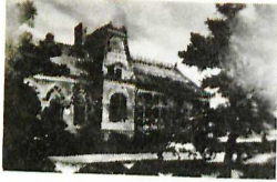
BUILDINGS ON A CLIFF WS-1925. LU.
