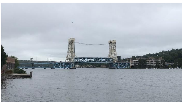
Figure 4. Hancock-Houghton Lift Bridge
