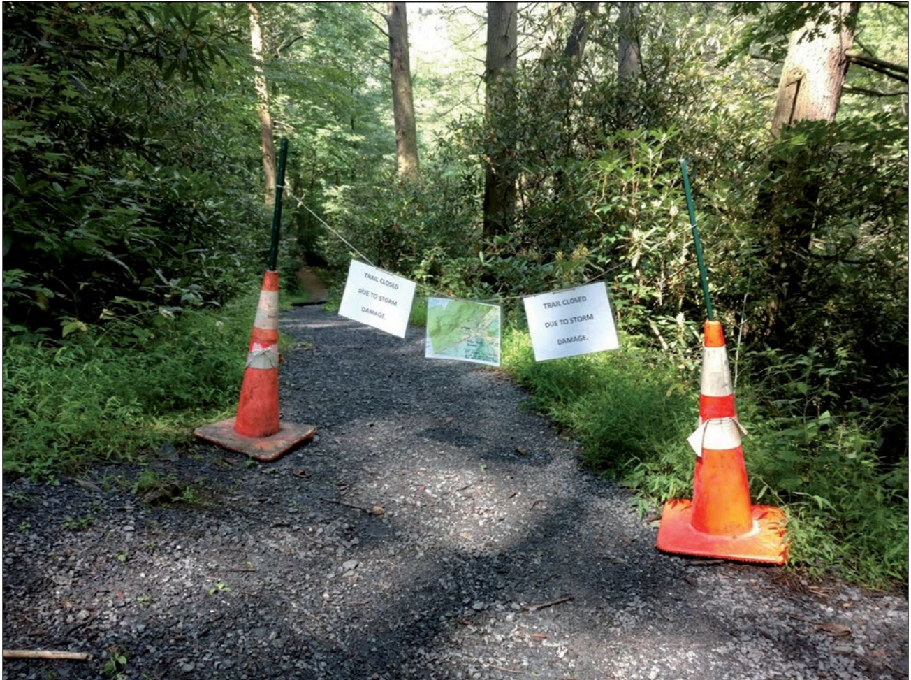
Aftermath of a rain storm that damaged a section of the Appalachian Trail in Pennsylvania. Such extreme events are not well modeled in climate projections. Photo by Patricia Leopold, Northern Institute of Applied Climate Science and Michigan Tech, used with permission.
