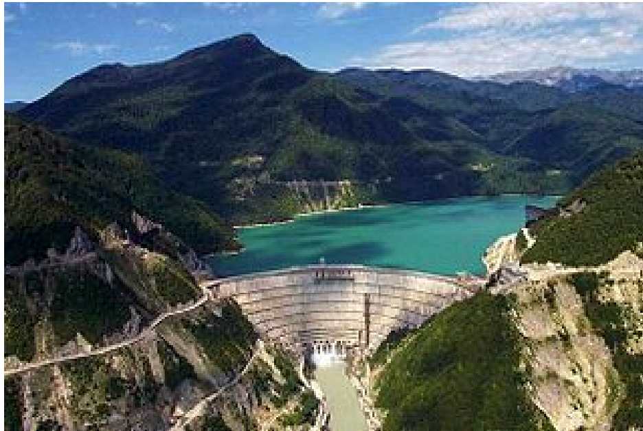
Figure 1: Enguri Dam looking north (source: https://en.wikipedia.org/wiki/Enguri_Dam )
